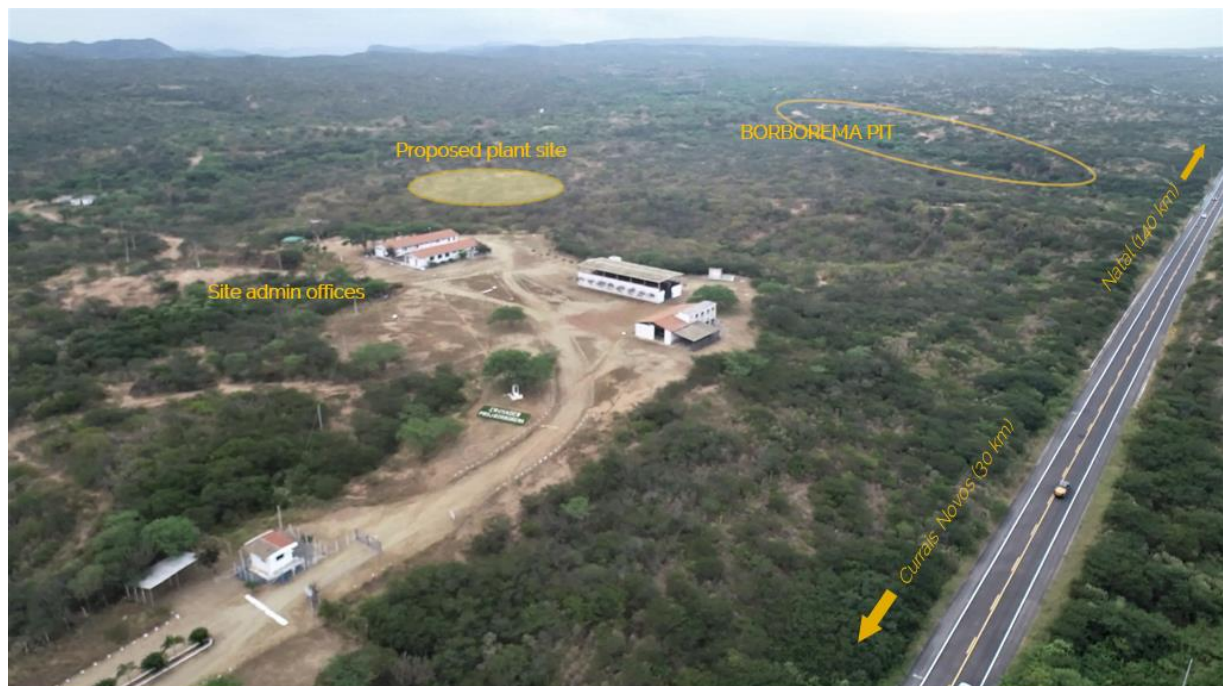
Figure 2. View to the east over the Borborema project site
