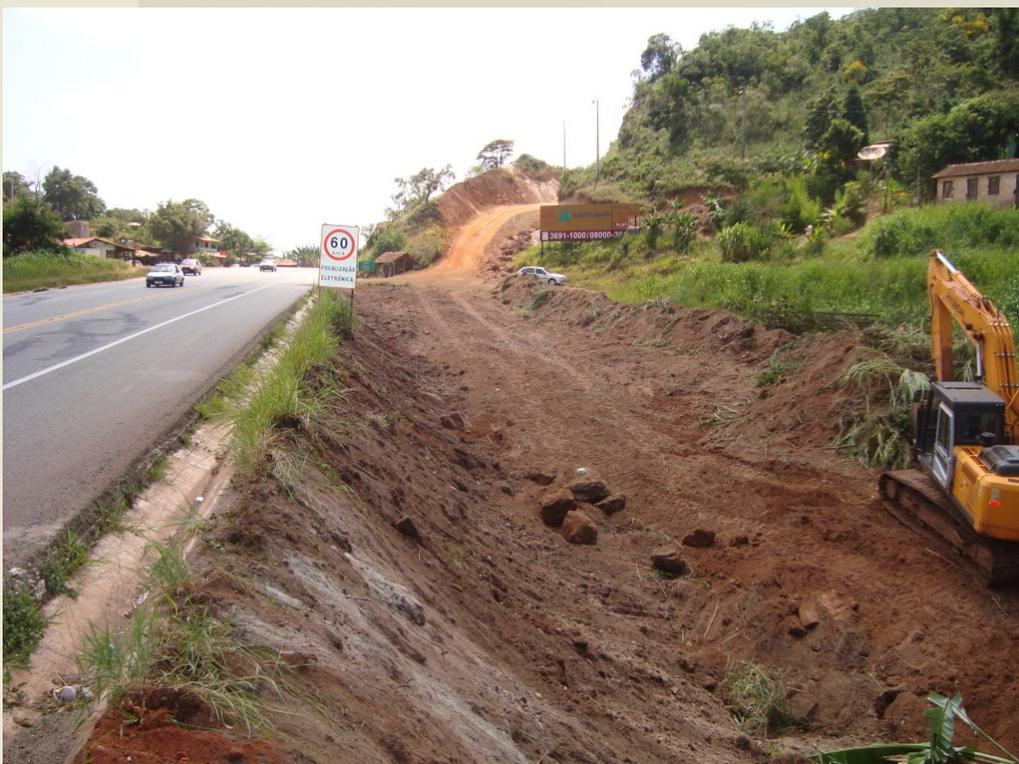
Photo 1: Clearing underway for access to Posse Iron Project
