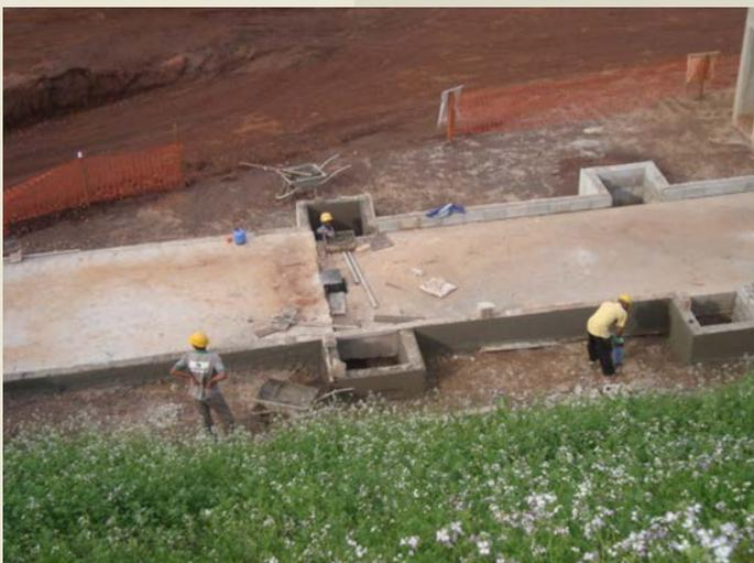
Figure 2: Weighbridge construction nearing completion
