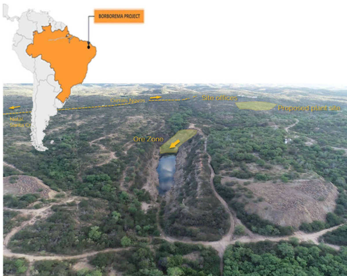
Figure 1. View to the south west over the Borborema pit showing the exposed ore zone and infrastructure.
